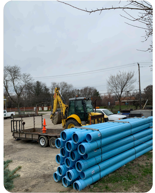
Lathrup Village DPS yard (Giffels Webster, 2020)
