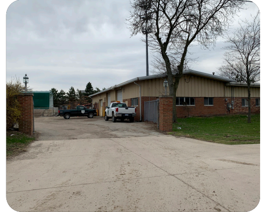
Lathrup Village DPS yard (Giffels Webster, 2020)
