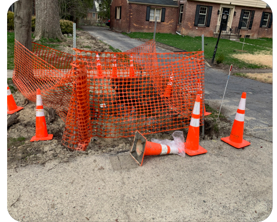
Drainage ditch repair (Giffels Webster, 2020)
