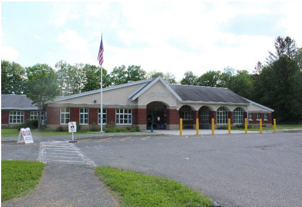
Lanesborough Elementary School.
