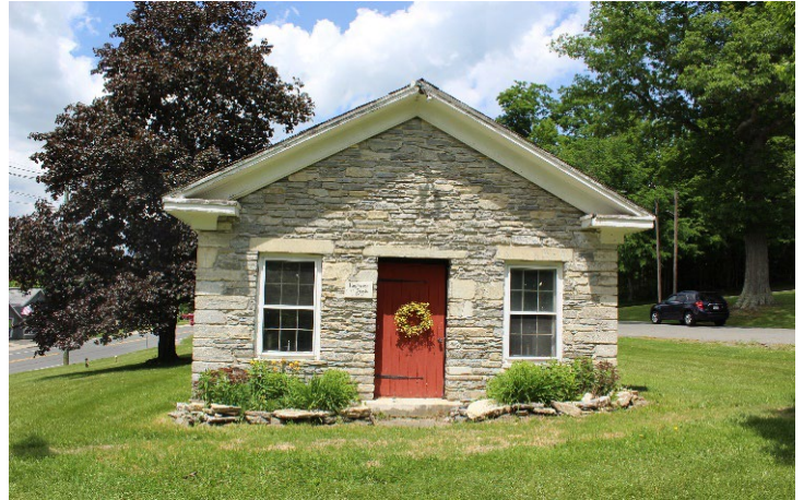
The original Northern Berkshire Registry of Deeds building on Prospect Street remains standing.
