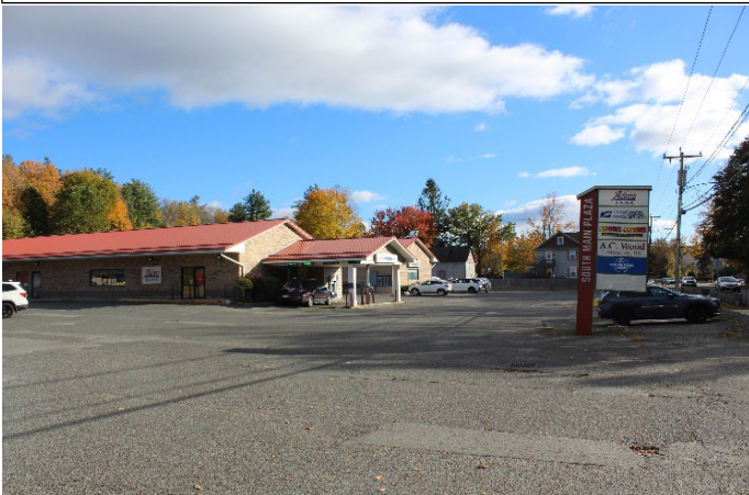
Figure 3.1 Commercial Plaza on Route 7 with current temporary police department facility
