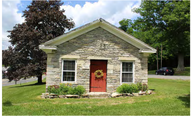
The original Northern Berkshire Registry of Deeds building on Prospect Street remains standing.
