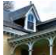
2 story porch supported by chamfered posts with arched brackets
