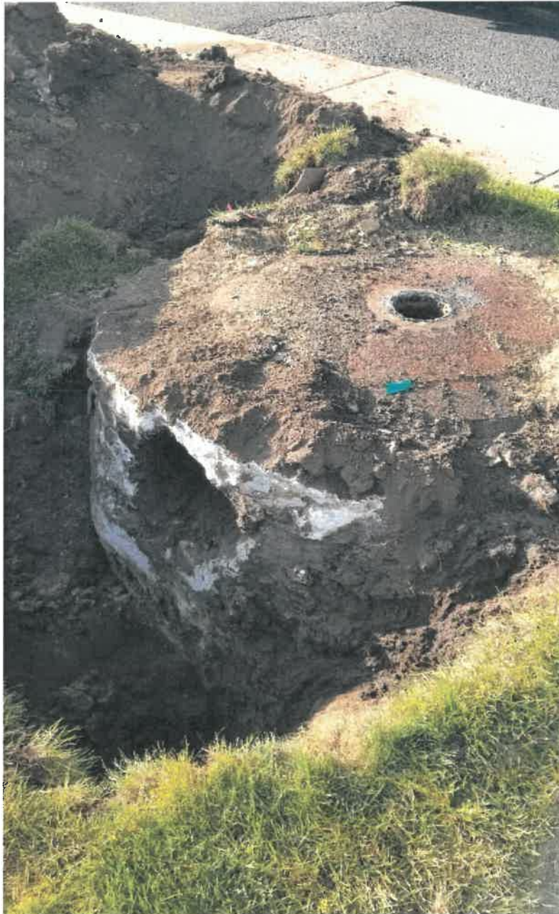
Existing footing that had supported the flagpole.
