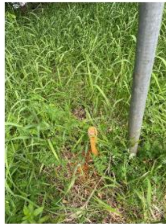
Piezometer - LDS Abutment
