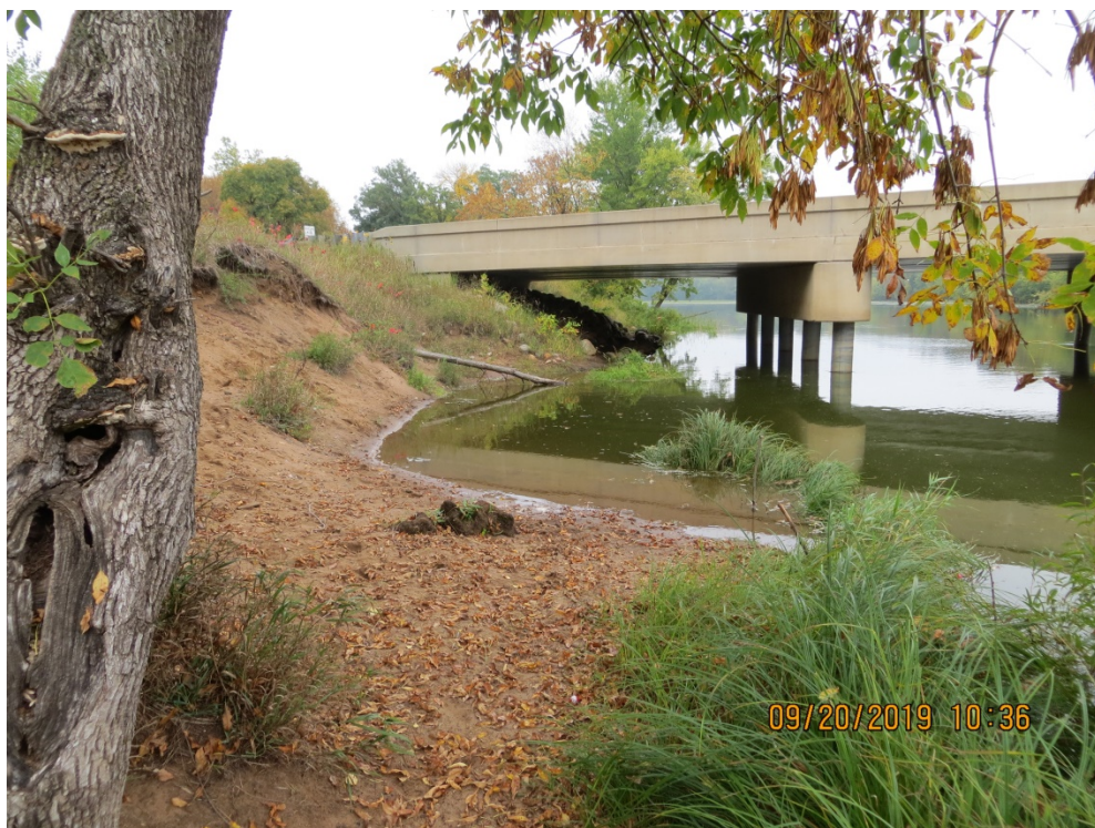
Above: Bank erosion along the Ann River – Fish Lake Shoreline looking east along the eroding bank towards MN 65.
