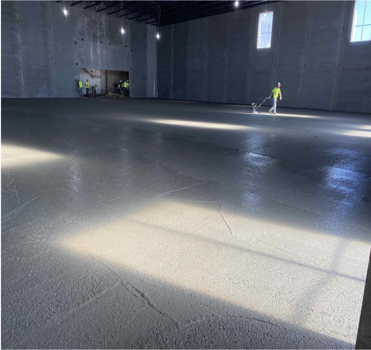
Concrete Poured at the Gym Floor
