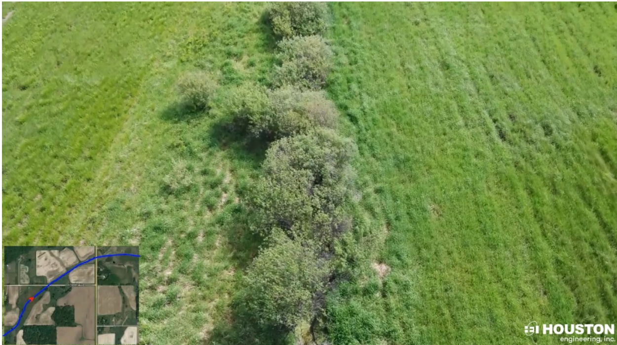
Photo 7: Tree growth within the banks of Branch 1 located at STA 42+00.
