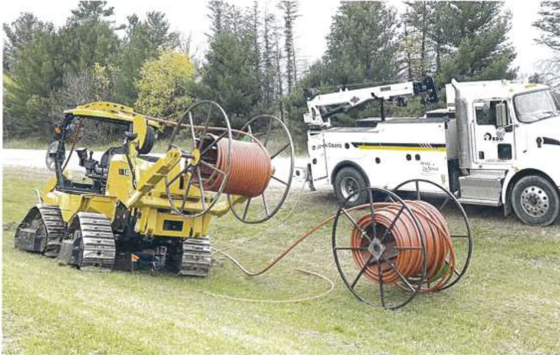
Fiber optic cable is being buried north of Mora along Highway 65 for a Midco expansion.
