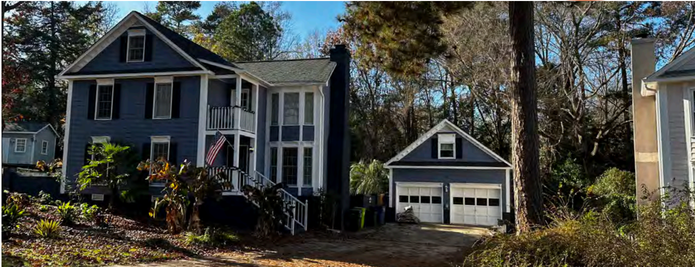
The Friarsgate neighborhood has a variety of housing types and styles. Many homes are well kept, although code enforcement issues do arise due to the age of some homes.
