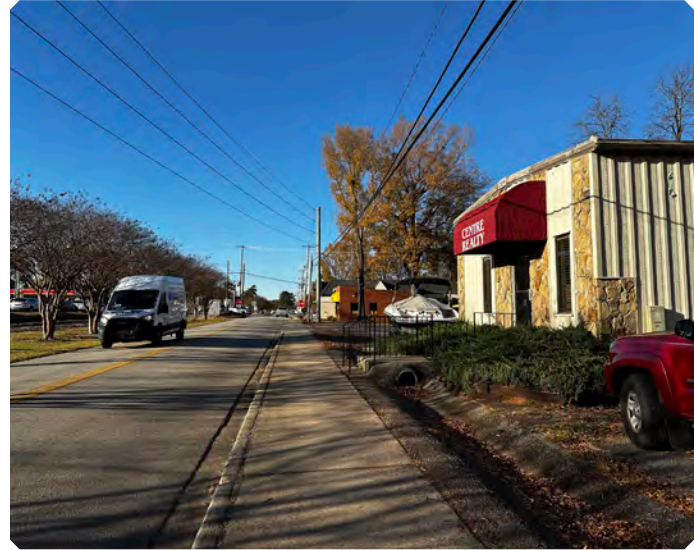
Woodrow Street functions as a key vehicular and pedestrian corridor near the center of Irmo. Currently sidewalks are narrow and only along a portion of the roadway.
