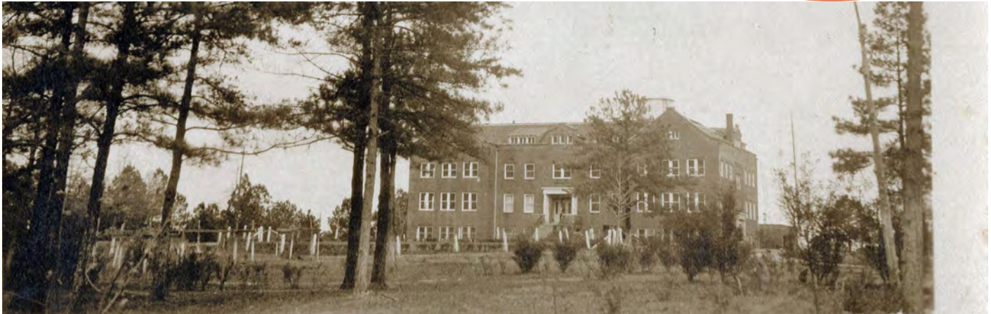
Former Administration Building at Harbison Agricultural College
