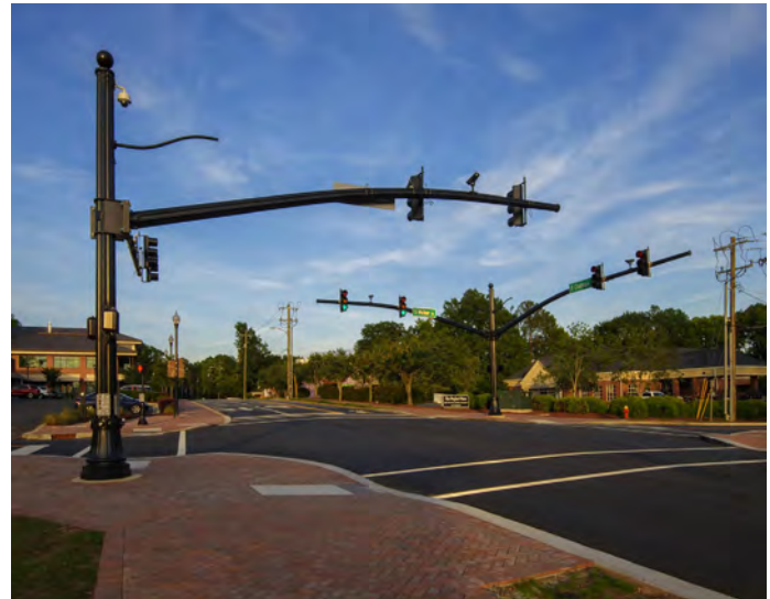
Mast arms could be paired with burying of utilities to reduce visual clutter in key areas of Town.
