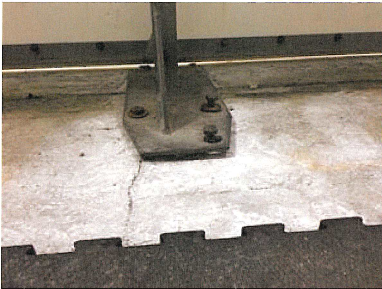
Anchors backing out, and footplate bent. This condition is evident in several locations.
