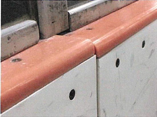
Uneven cap rail, resulting effect of an uneven substrate.
