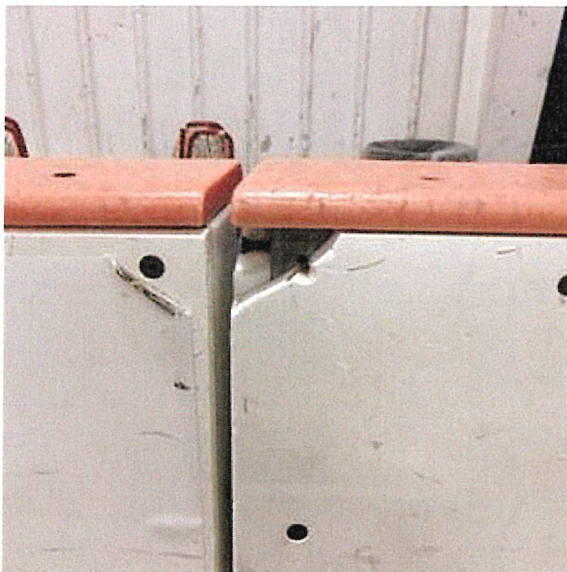
Typical condition. Broken HDPE facing and gaps in facing.
