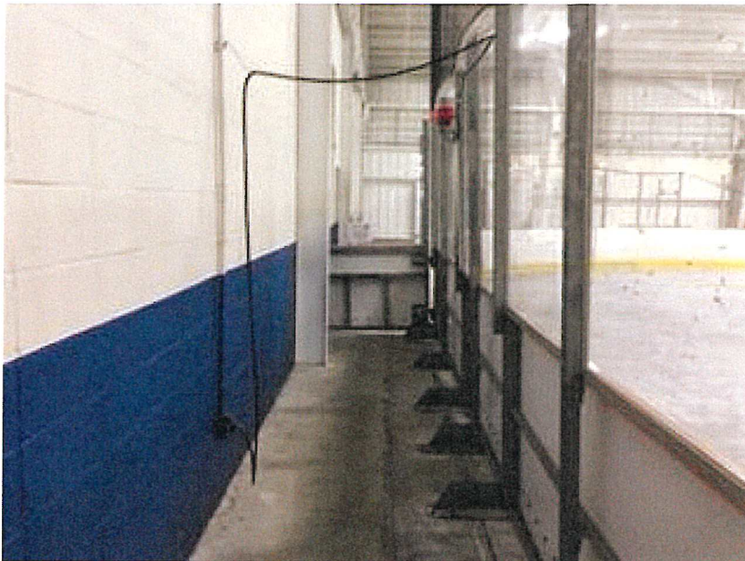
Weight of equipment gate is causing gate to sag, and difficult to close properly.
