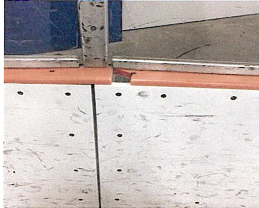
Another area with missing/broken HDPE creating a hazard.
