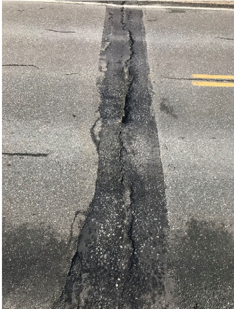
Joint 3 over Pier 3
