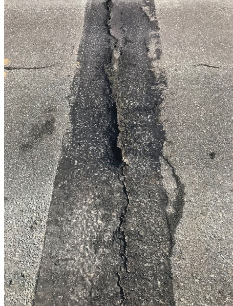
Joint 3 over Pier 3
