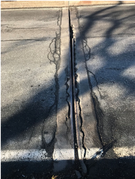
Joint 5 over Pier 5
