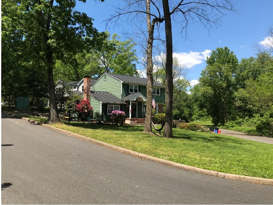
View of existing front porch to be removed for new front porch addition.
