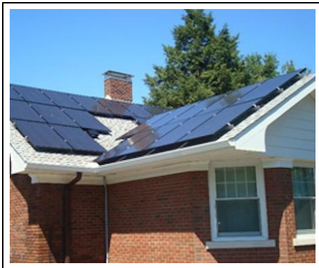
Roof Mounted Solar
