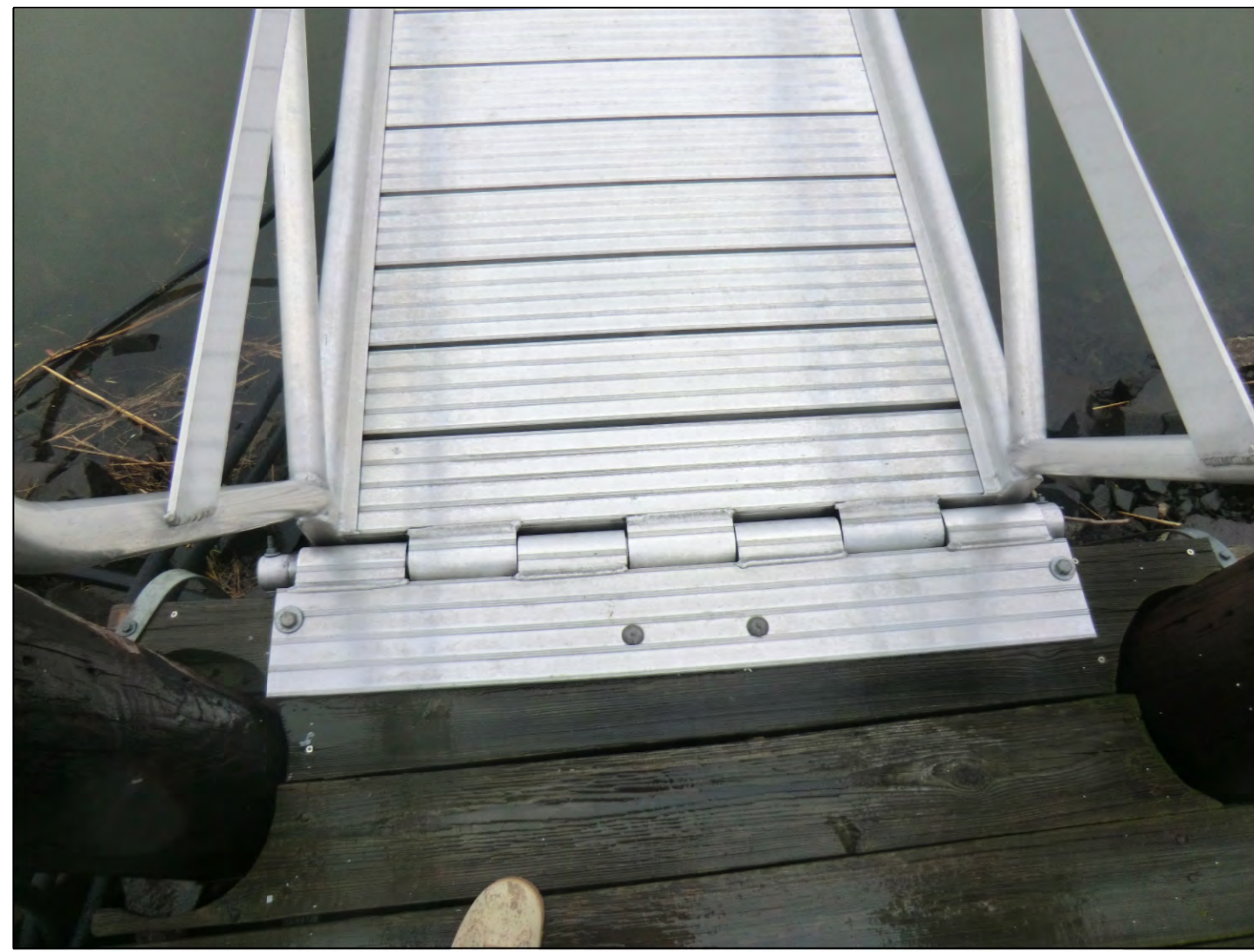
TYPICAL ACCESS RAMP BOLT CONNECTION NTS
