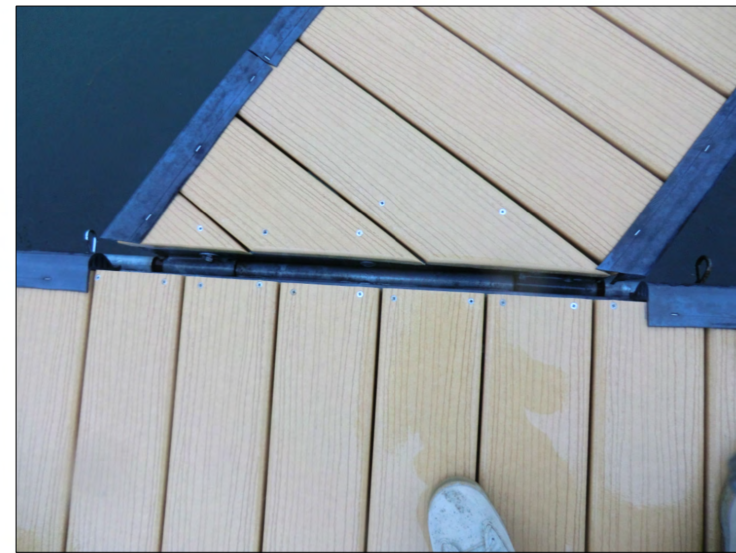
TYPICAL DIAGONAL PIER HINGE CONNECTION NTS
