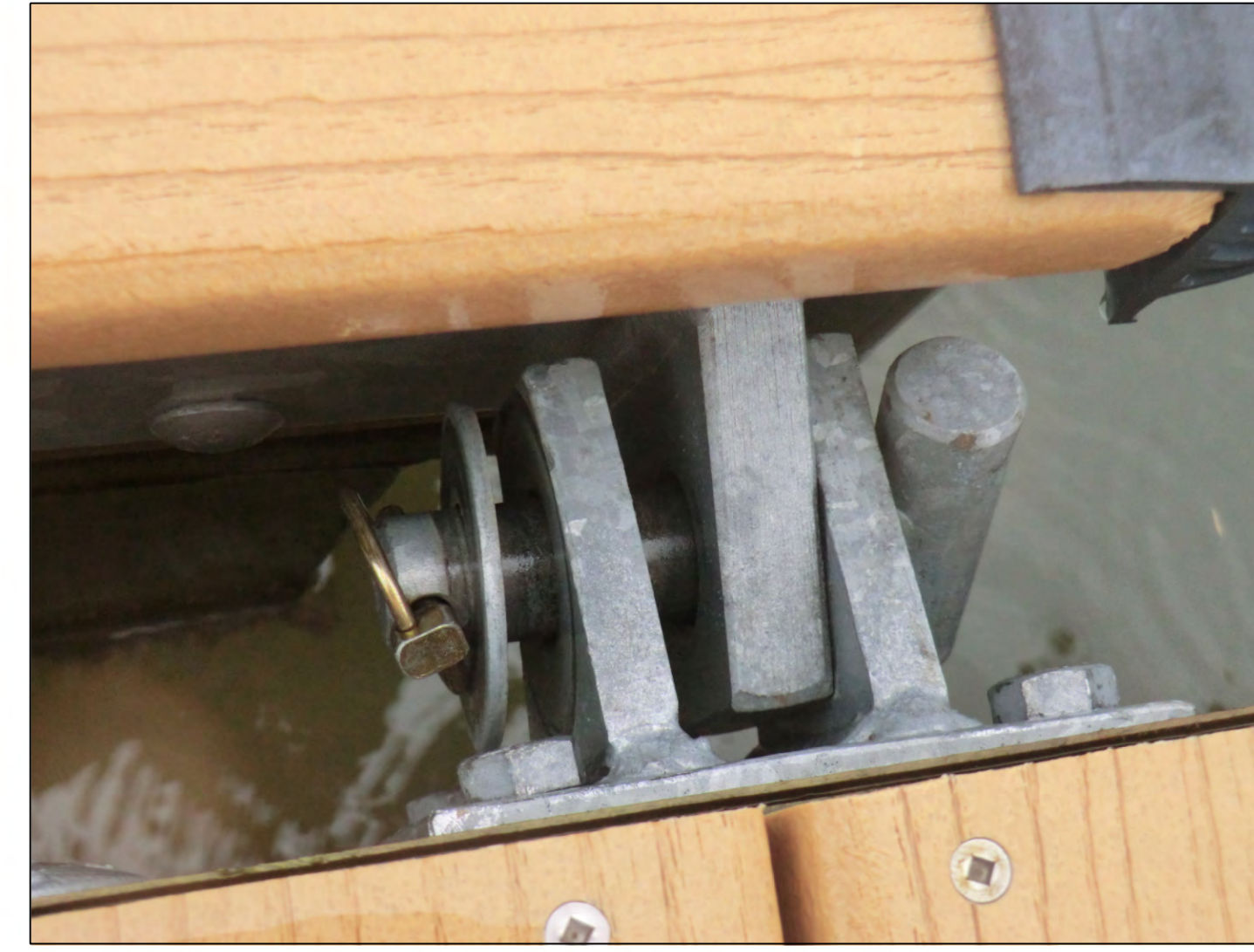
TYPICAL STRAIGHT PIER HINGE PIN CONNECTION NTS
