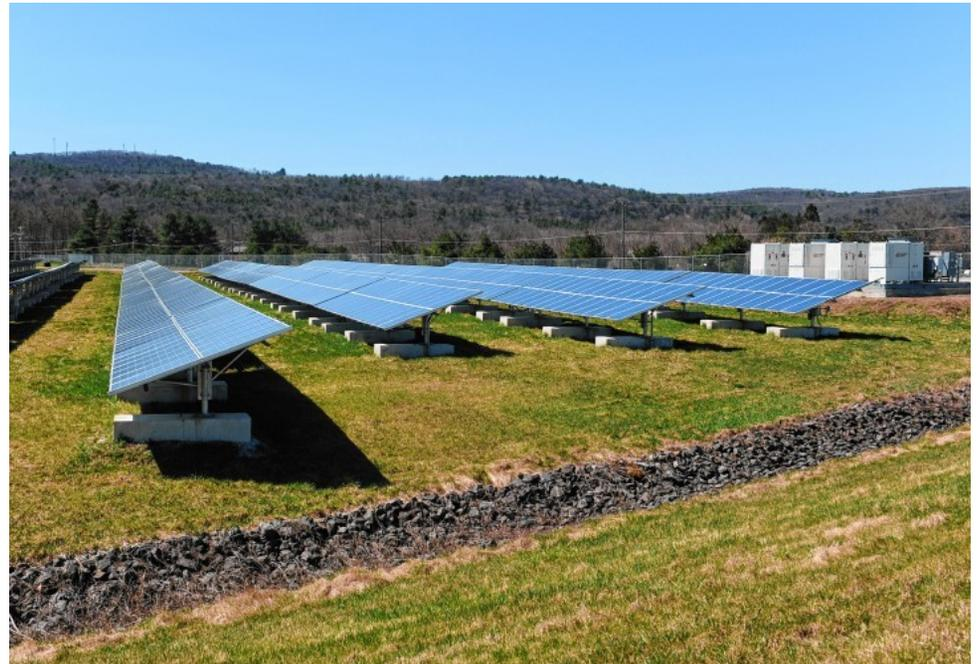
*A 2MW solar array on the City's capped landfill has been in operation since 2012 and generates equivalent to half of the municipality's energy use.*
