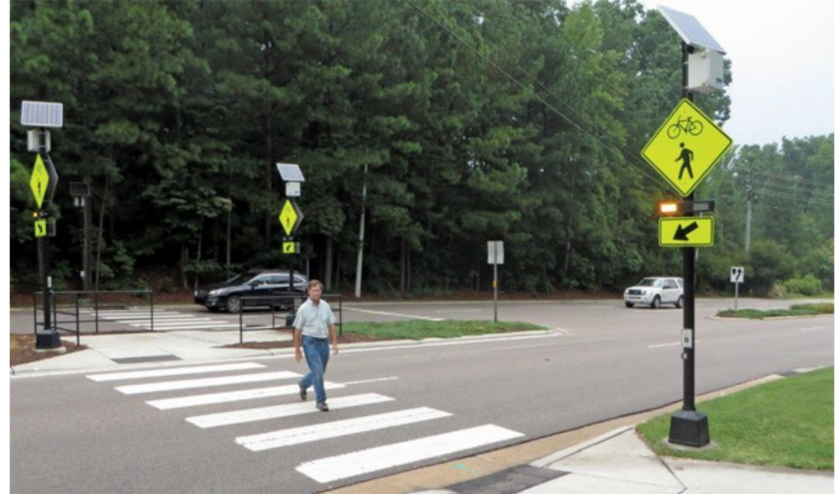
Long crosswalk across 4 lanes with better safety features (Cambridge)
