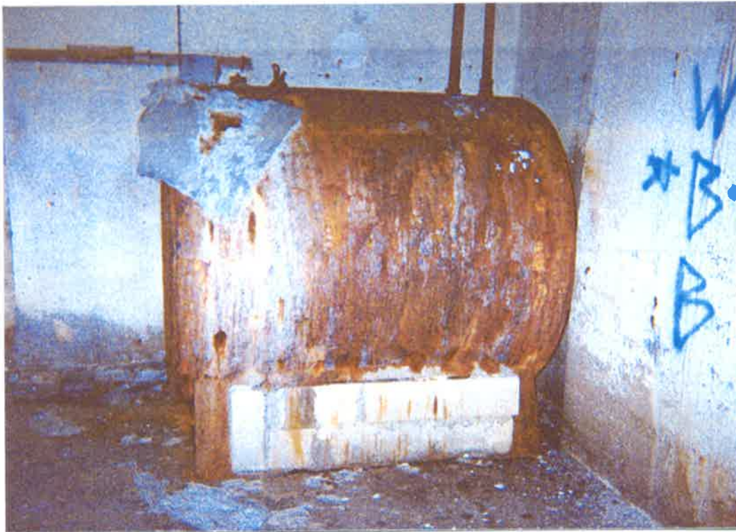
Photograph 3 – AST located in basement
