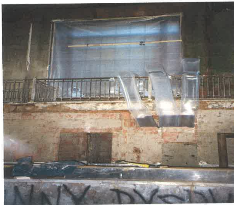
Figure 6-Former bank area during remediation
