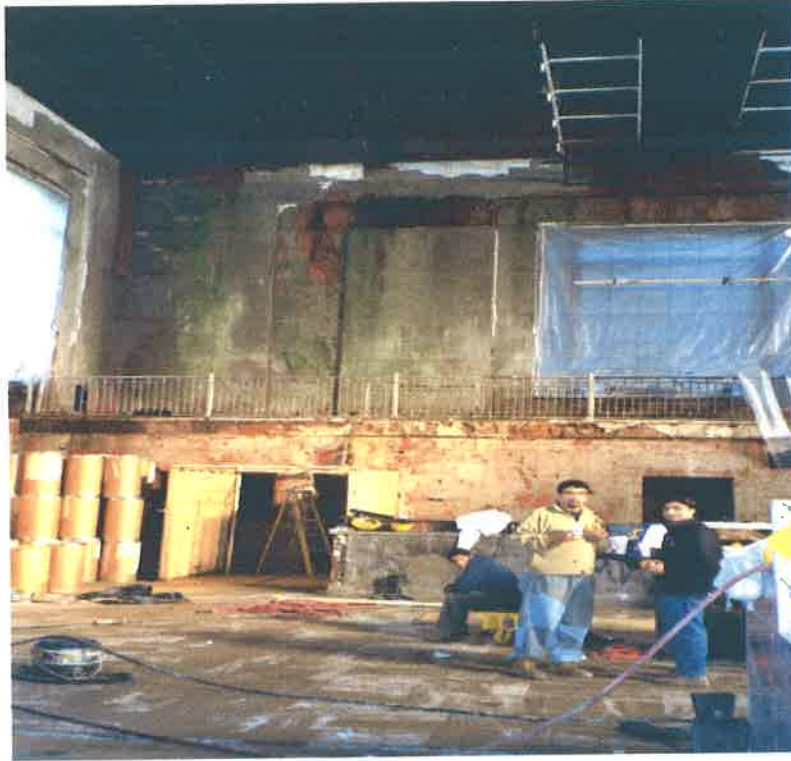
Figure 5-Former bank area during remediation
