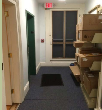
Accessible route to the elevator in library has obstructions.
