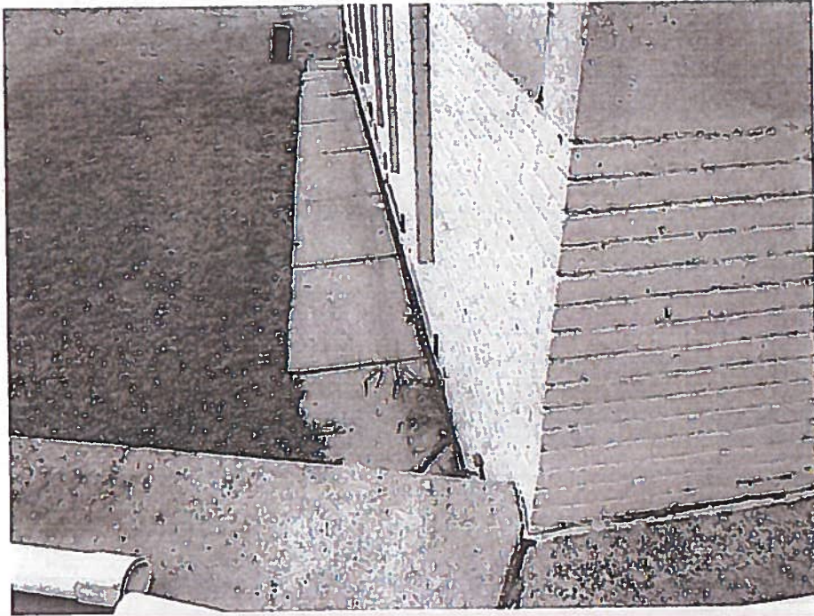
Subsiding and ajar cement slabs at base of west wall (Note missing sealant in slab/wall junction)
