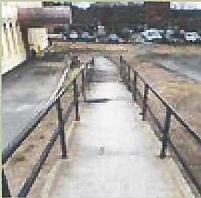
The library's accessible entrance ramp has cracks and crevices. Route from parking to entrance crosses an emergency vehicles lane.
