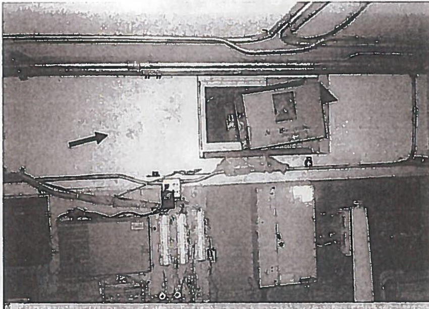
Water Damage to Foundation Wall
