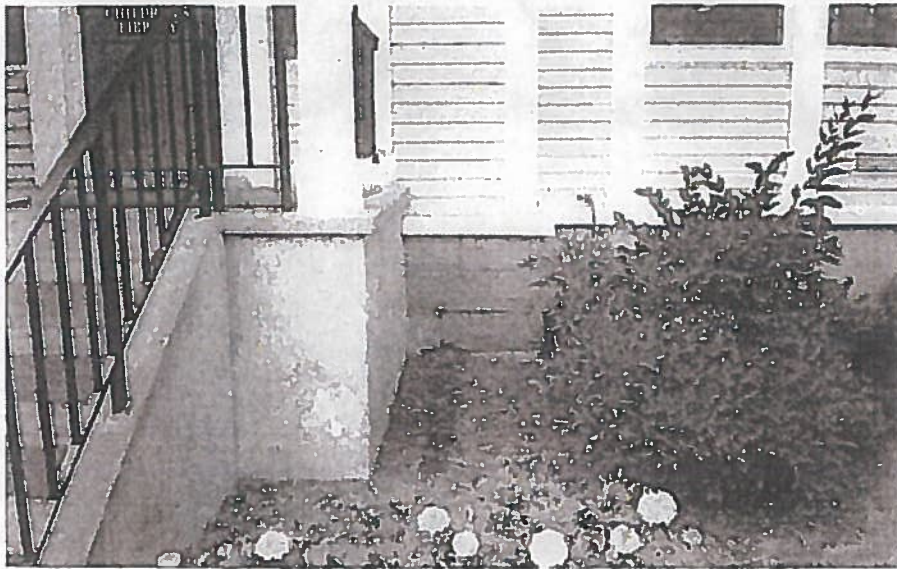
Pooling Rainwater from Roof, Note Damage to Foundation Stone in Proximity to Pool
