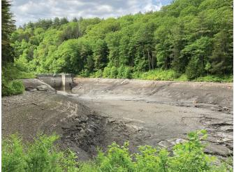
The water is contained with a dam and crest gate. The crest gate allows us to raise or lower the water level approximately three feet.
