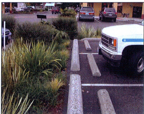
Bioinfiltration methods such as planted islands capture stormwater from parking areas, reduce non-point source pollution, and provide landscaping within these areas.
