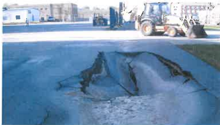
Stormwater System Collapse on Court Street in 2014
