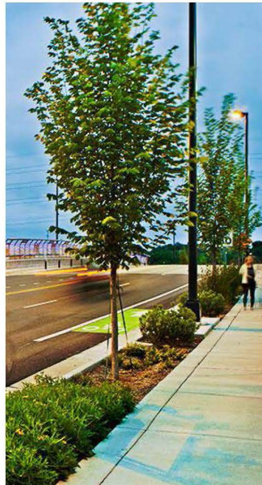
Contiguous Bioswale along Northwest Highway Provides a Green Edge between Pedestrian and Vehicular Traffic
