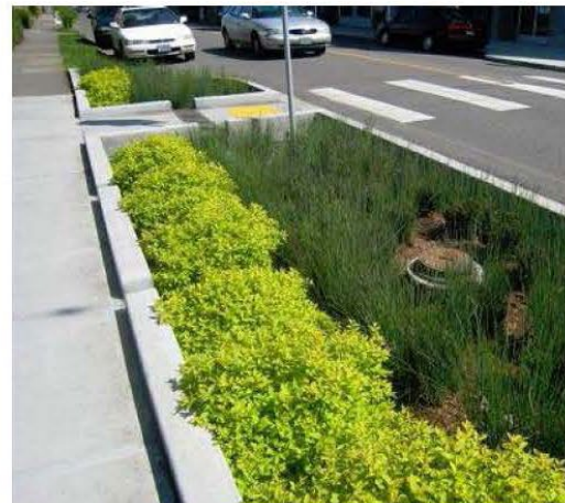
6" Curbed Depressed Bioswales "River" Serve as Parkways Filtering Run-off before Releasing into the Watershed
