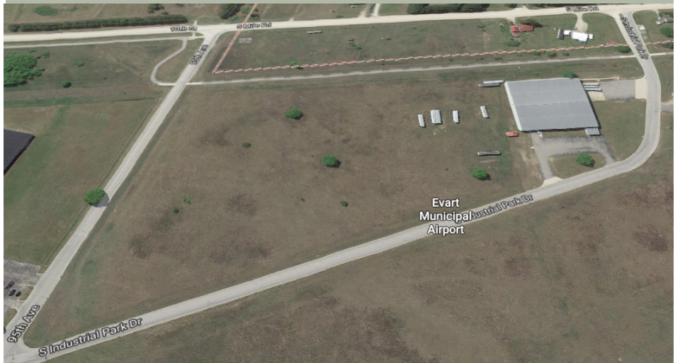
Evert Air Industrial Park, parcels on the southern side of the tarmac
