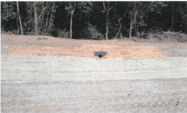
Top Left: Eroded hole one. Bottom Left: Earth fill, diversion, and drop outlet completed on hole one.
