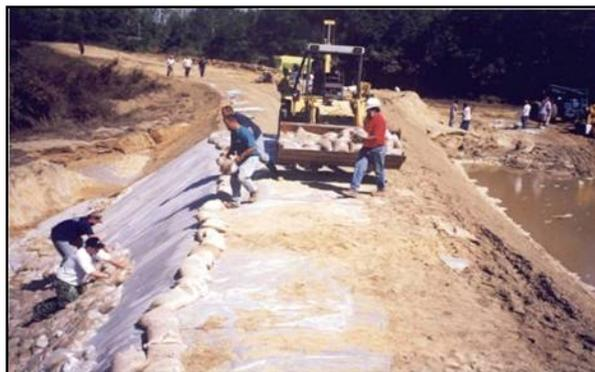
**Figure 1.6: Dike Repair after Hurricane Floyd, 2000**
