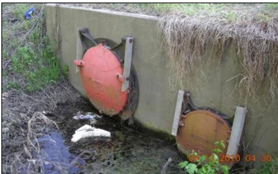
*Figure 1.9: Flap Gate Backflow device on culverts*
