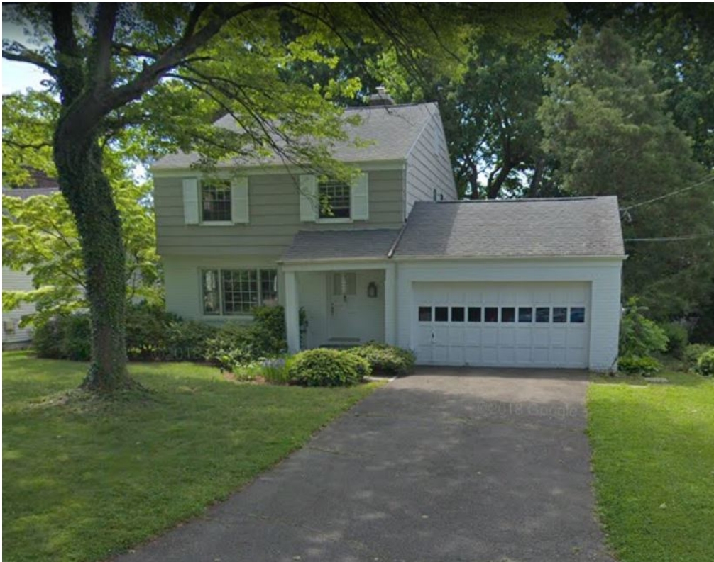
P-110 NORTH ROAD : 79.B/3/22 CATHERINE VERGARA
