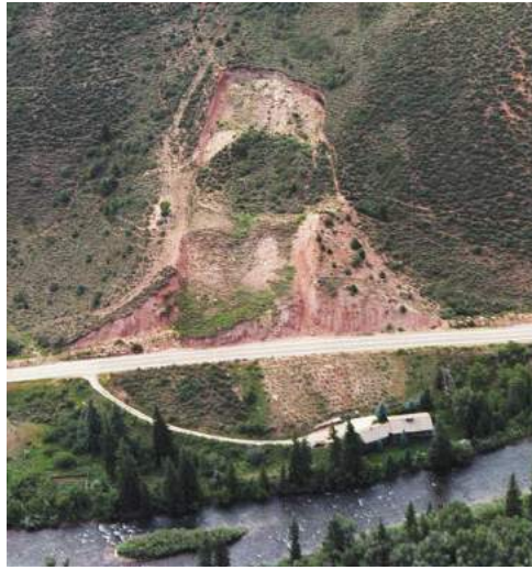
House built in a flood plain at the toe of a landslide near Wolcott. Photo by D. Noe
