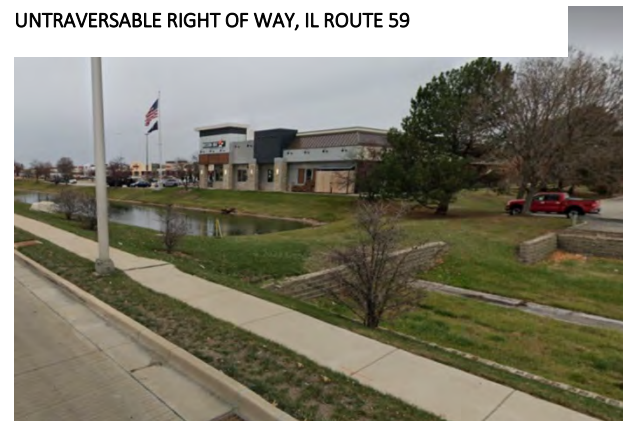
UNTRAVERSABLE RIGHT OF WAY, IL ROUTE 59
