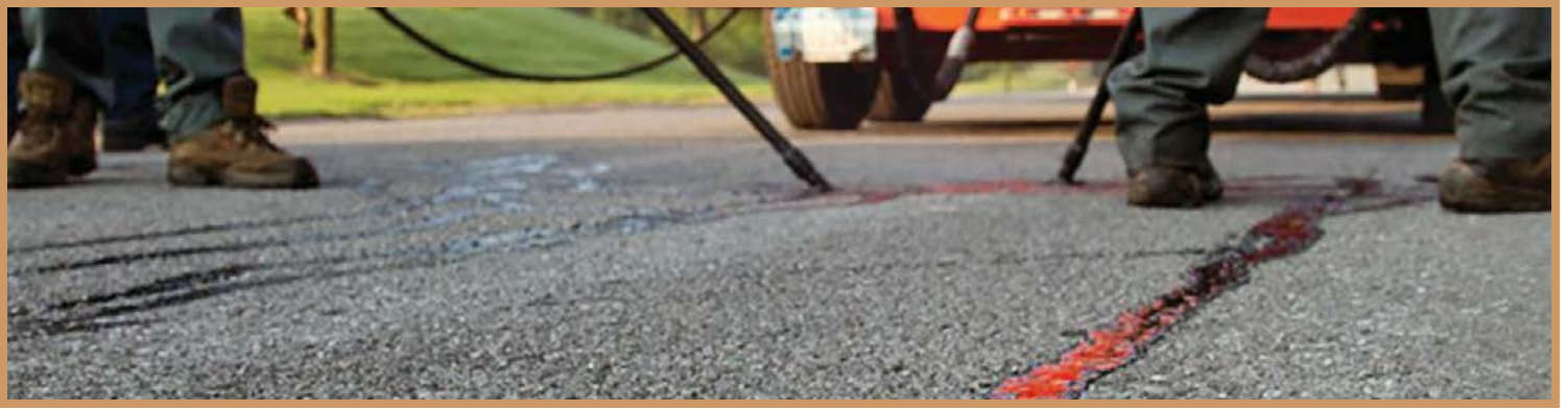
How to Crack Seal, Source: AsphaltPro Magazine
