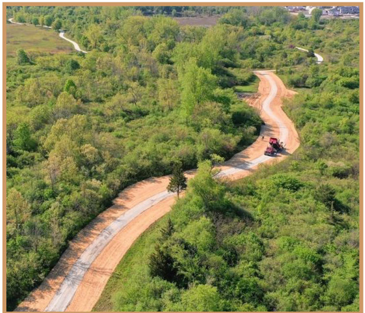
New Trail in Danada Forest Preserve, Source: Daily Herald
