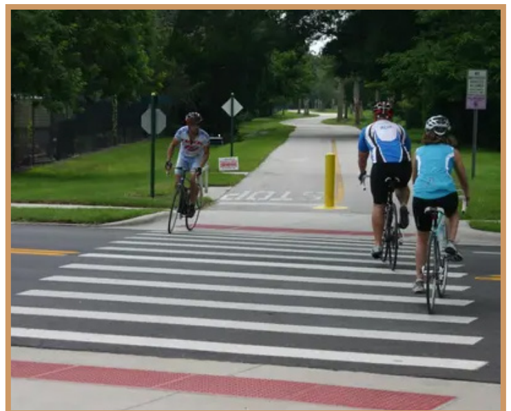
Road Crossing, Source: American Trails
