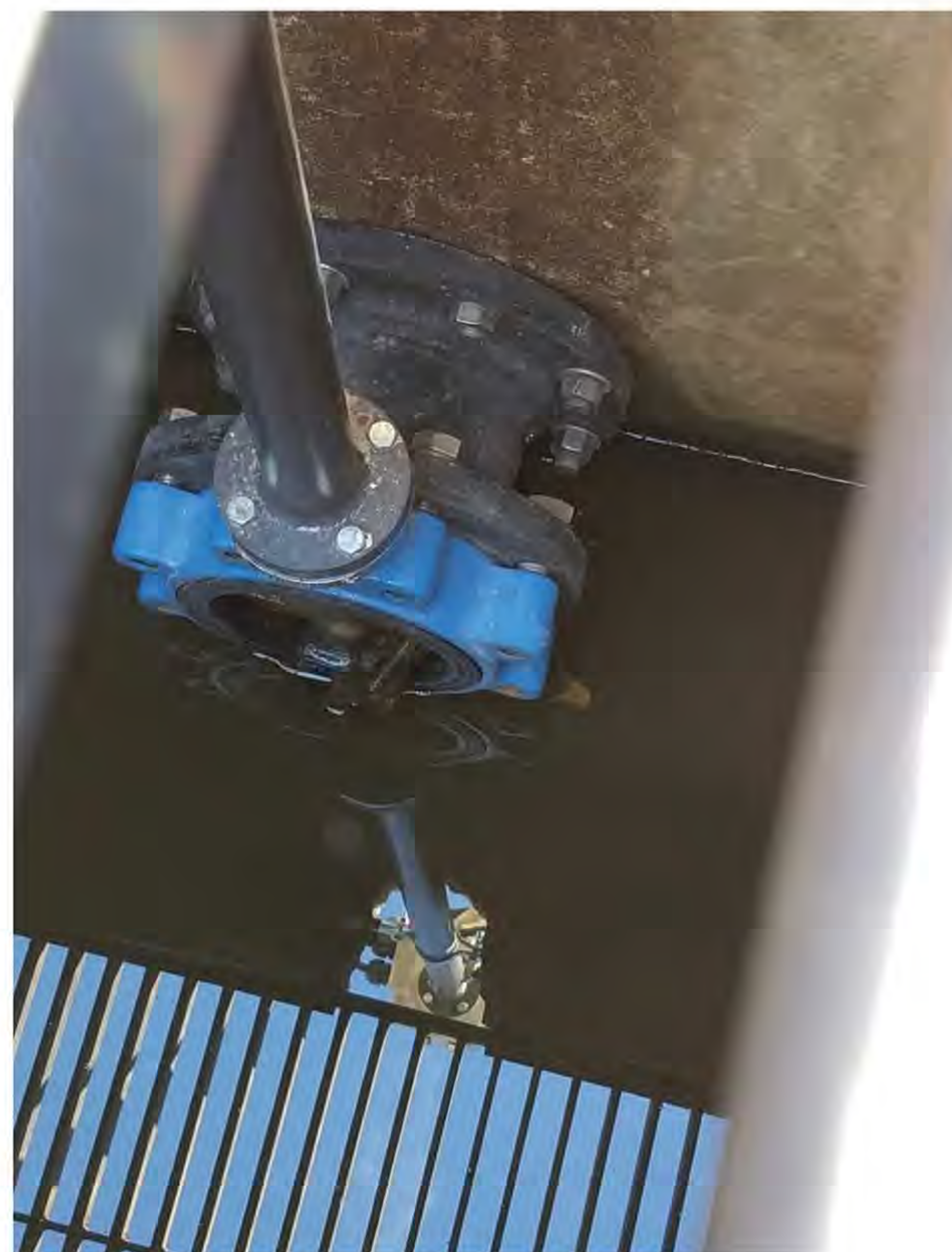
The continuous monitoring and adaptive control system uses the water-level data along with storm forecasts to determine the optimal percentage that the outlet's discharge valve should be open to minimize flows to the combined sewer. OptiRTC
