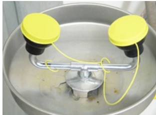
Figure 2. Eyewash with protective covers.
