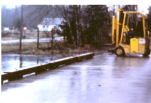
A bull rail at an unused edge of a dock reduces the risk of a forklift wheel slipping off.
