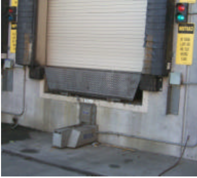
Dock mounted vehicle restraint clamps to a bar under the truck.
