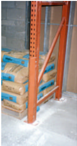
Rack leg is reinforced against forklift damage
