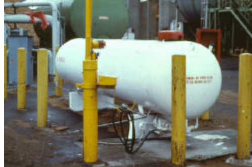
Propane tank used to refill the forklift LPG tank is protected against vehicle damage by heavy posts.
