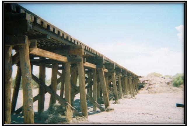
It is important to note that no drilling, sounding or excavation was performed during this investigation. Also, conditions such as cracked stringers and pile pumping are frequently only evident while a train is traveling over the superstructure. There was no train observed during this field review.
