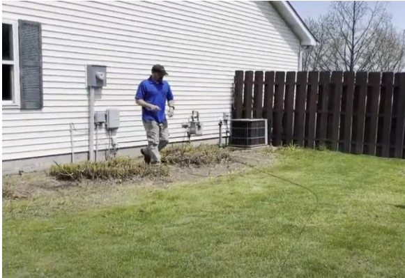
Running the fiber drop to the house
