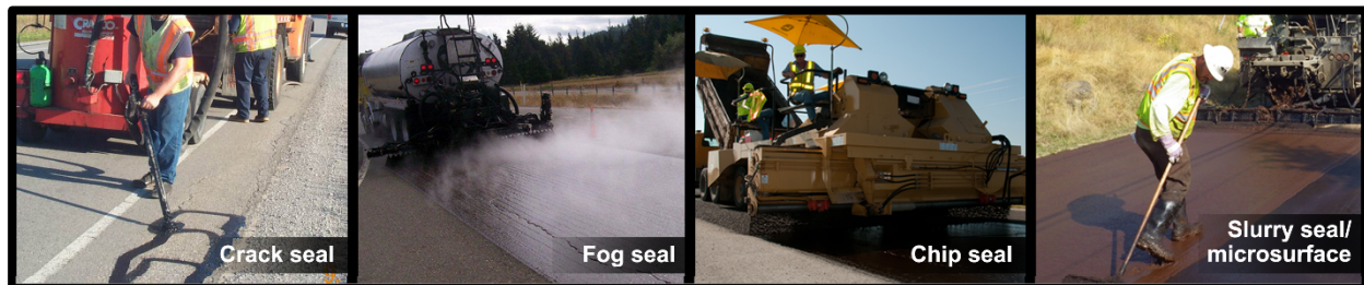
Figure 3: Examples of capital preventive maintenance treatments—(from left) crack seal, fog seal, chip seal, and slurry seal/microsurface.
