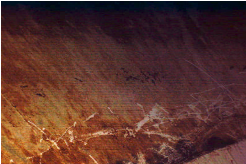
(54) Wet interior lower sidewall coating is in good condition, with mineral staining.
