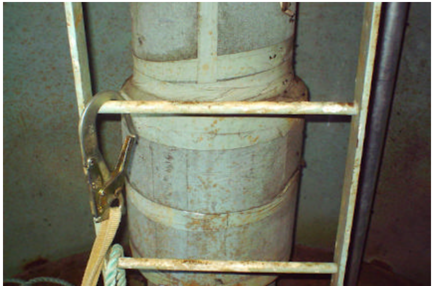
(36) Dry interior top platform - fill pipe penetration into wet interior.
