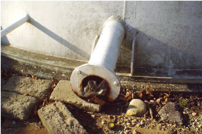
(16) Exterior condensate drain line - screen is not functional. Line is probably plugged.
