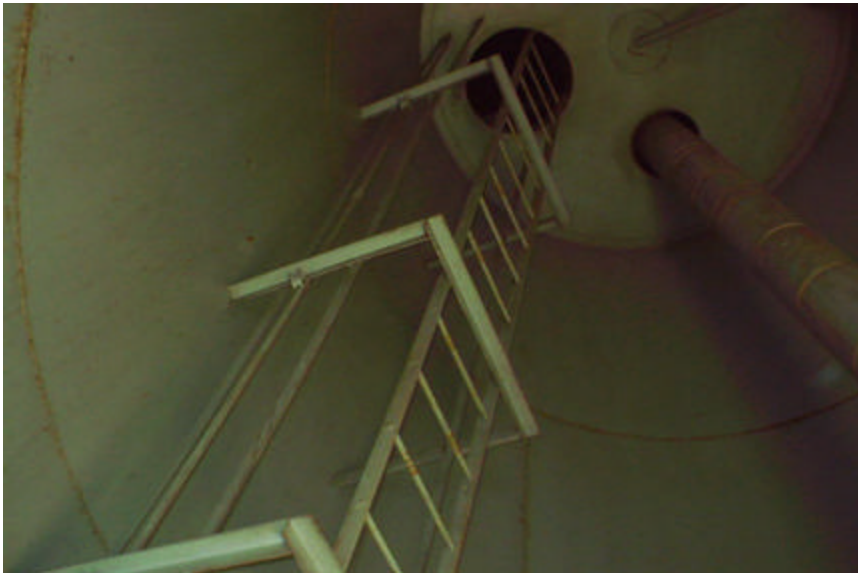
(22) Dry interior base cone coating is in good condition.
