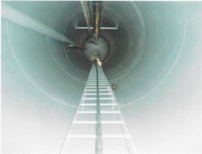
4) Riser section with no coating failures.
