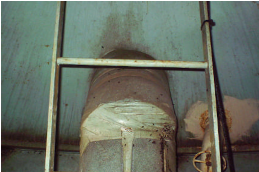
(37) Dry interior access tube - minor pinhole corrosion.
