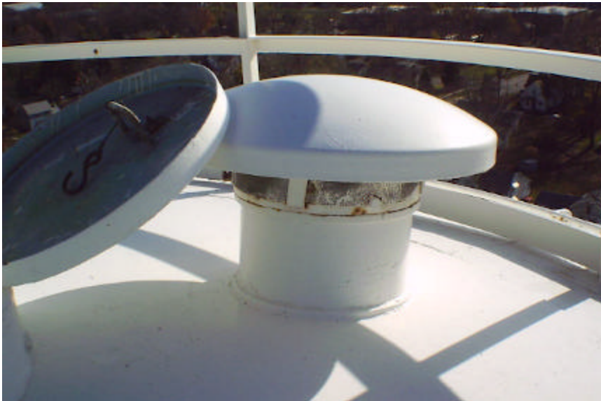
(43) Exterior roof vent screen.
