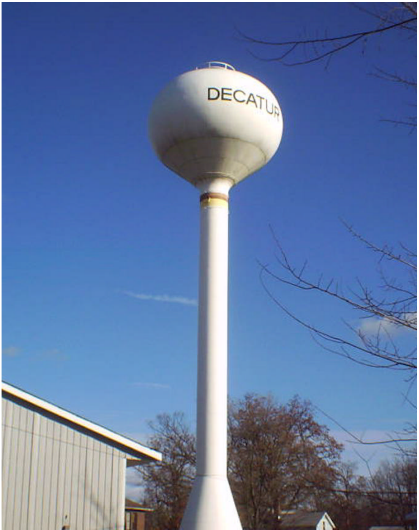
(1) 200,000 gallon water storage tank located in Decatur, MI.
