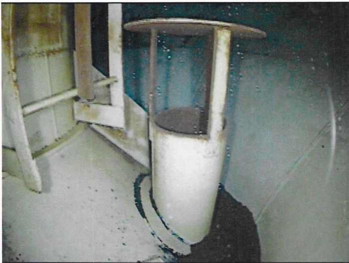
12) Bowl and cone section with no coating failures.
