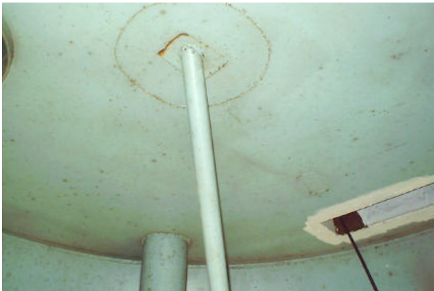
(25) Dry interior - bottom side of condensate platform. Antenna penetration no longer in-use.
