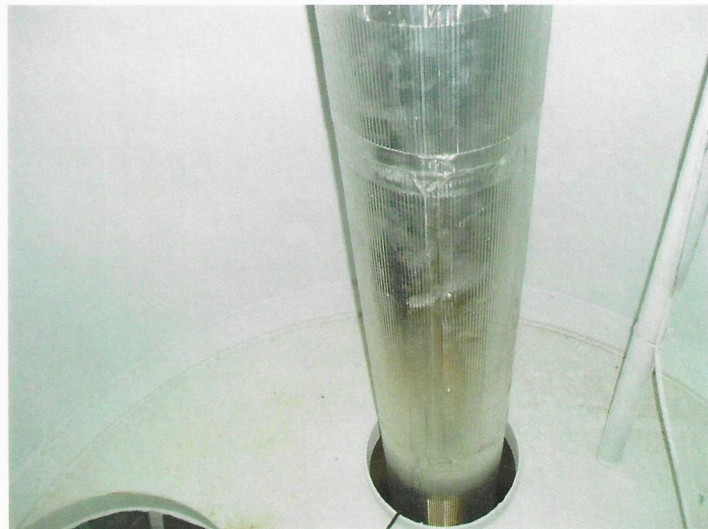
5) Typical fill pipe insulation cover is intact.
