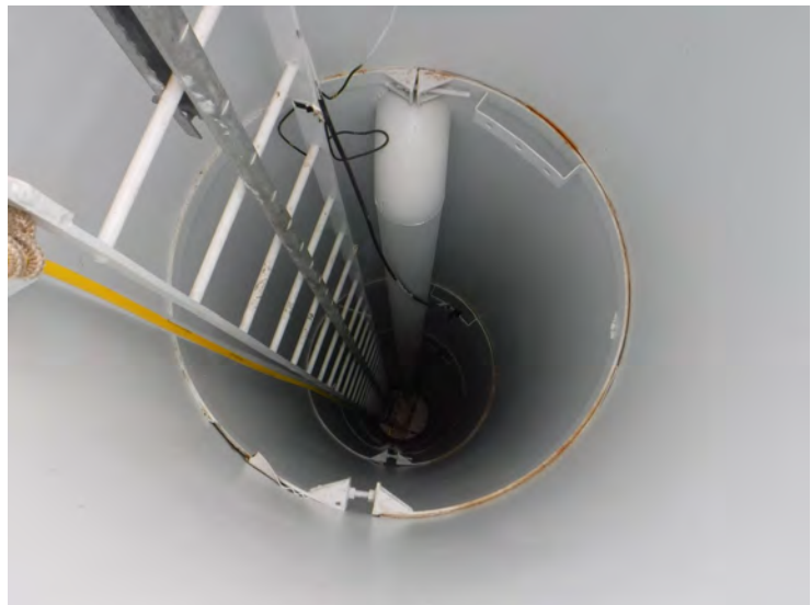
35) The access tube ladder is in good condition. The ladder is equipped with a fall prevention device.
