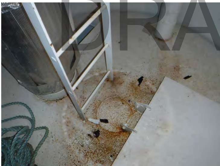
30) Minor coating failures on the top platform. The top platform opening and cover are in good condition.
