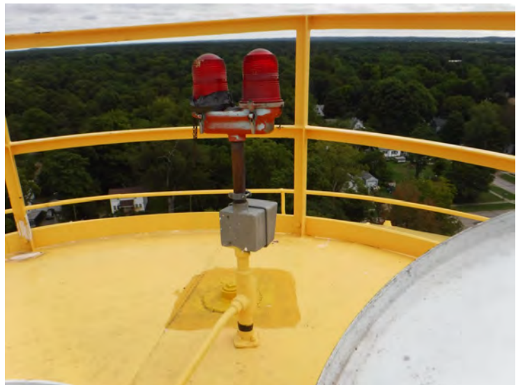
17) One of the aviation light globes is being held in place with electrical tape.
