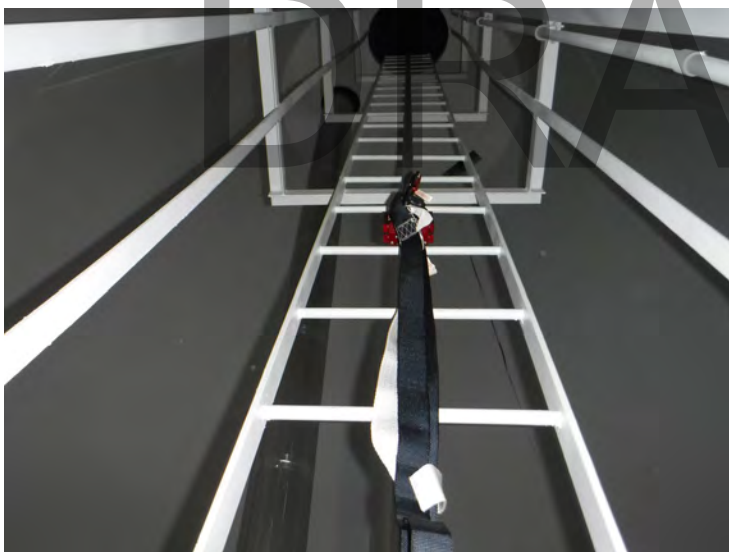
24) The basebell ladder fall prevention starts halfway up the ladder.
