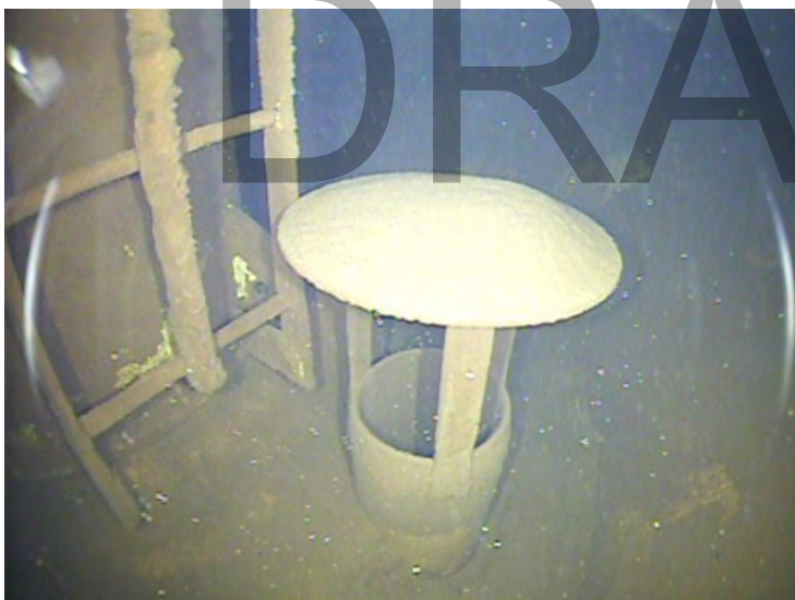
51) The fill/draw pipe is in good condition. There is a deflector plate at the end of the pipe.
