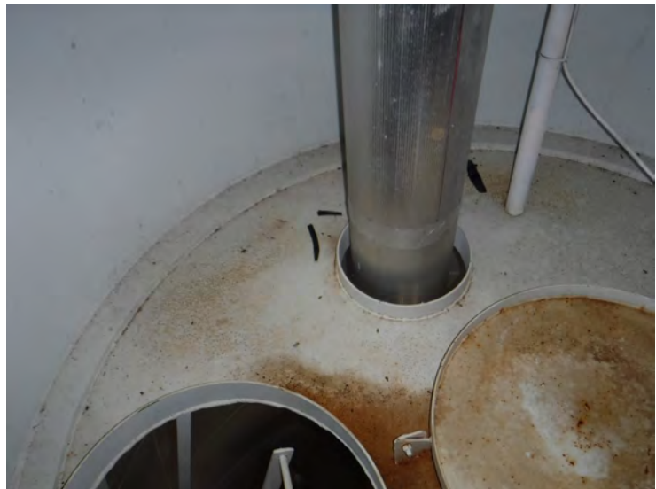
26) There is rust bleedthrough and a few minor spot failures on the condensate platform.
