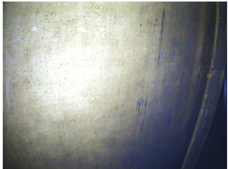
41) The sidewall coating is in good condition overall.
