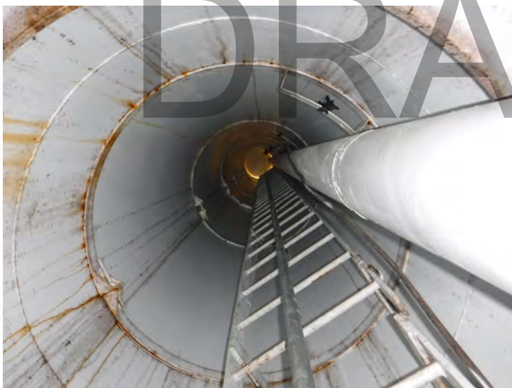
33) There is rust bleedthrough and streaking at the antenna cable attachment brackets in the access tube.
