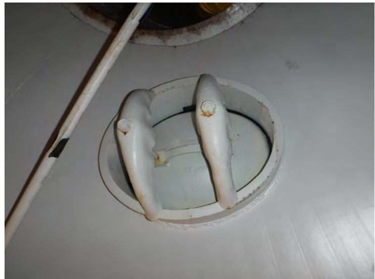
32) The wet interior manway in the transition cone is in good condition.
