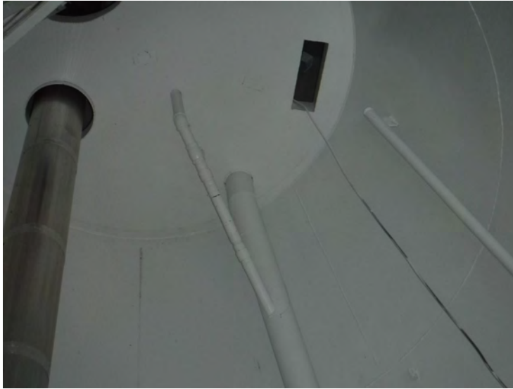
25) The condensate drain routes to the overflow pipe and is in good condition.
