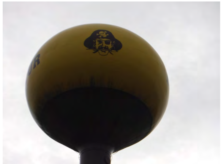
11) The sidewall coating is in good condition with no significant failures.
