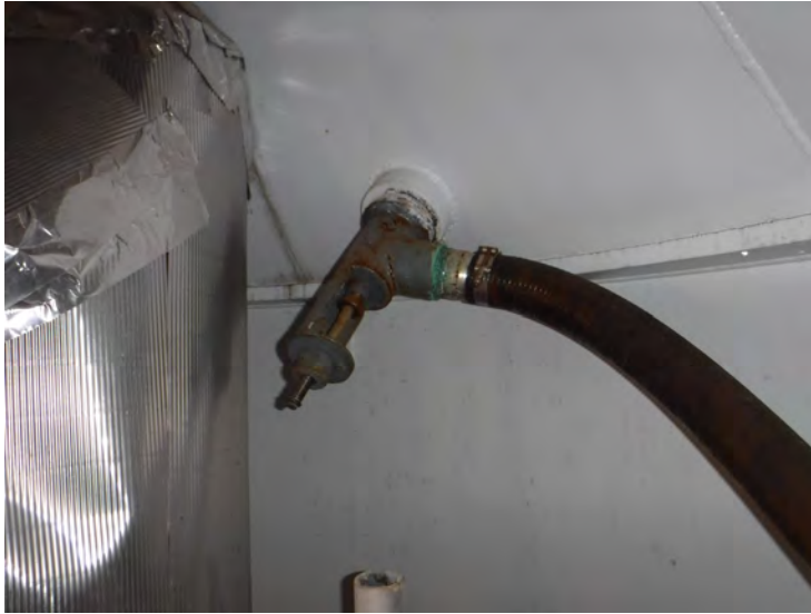
31) The mud valve appears to be in good condition.
