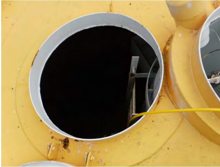
19) There is no gasket on the wet interior hatch.
