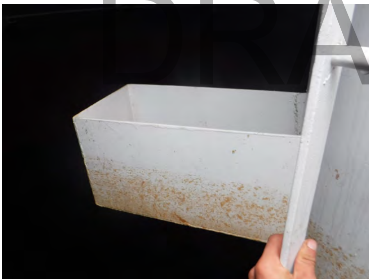
39) The overflow weir box is in good condition.
