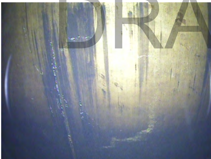
42) Pinhole coating failures on the sidewall.
