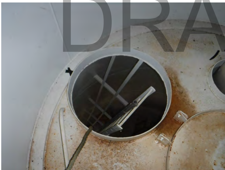
27) The condensate platform opening and cover are in good condition.
