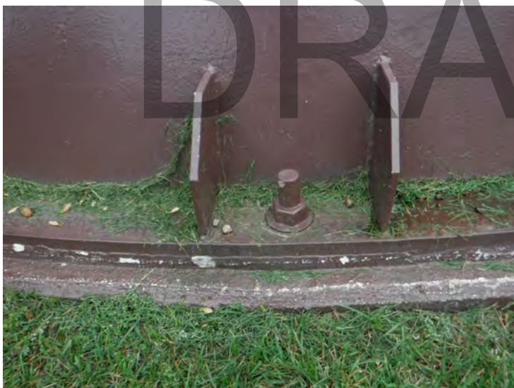
3) Typical anchor bolt is in good condition.
