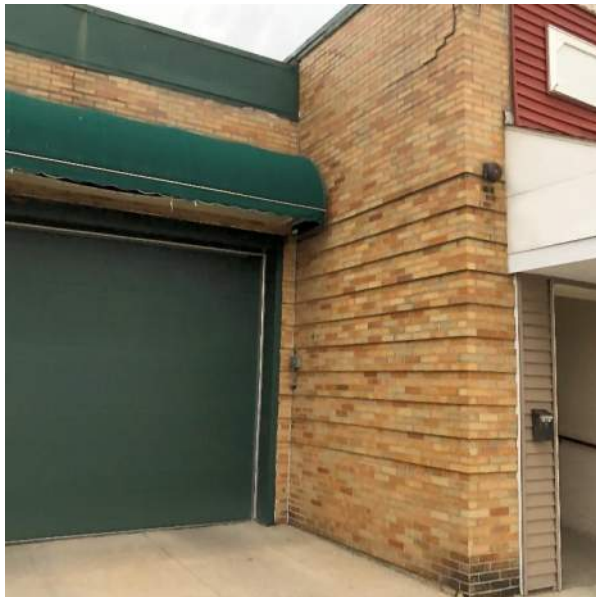
B-v: Failing Brick
