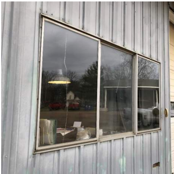
C-i: Broken panes of glass
