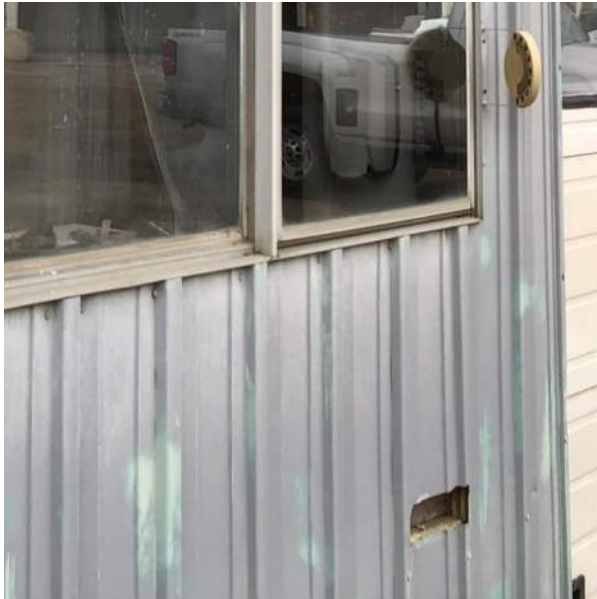
B-ii: Hole in Siding
