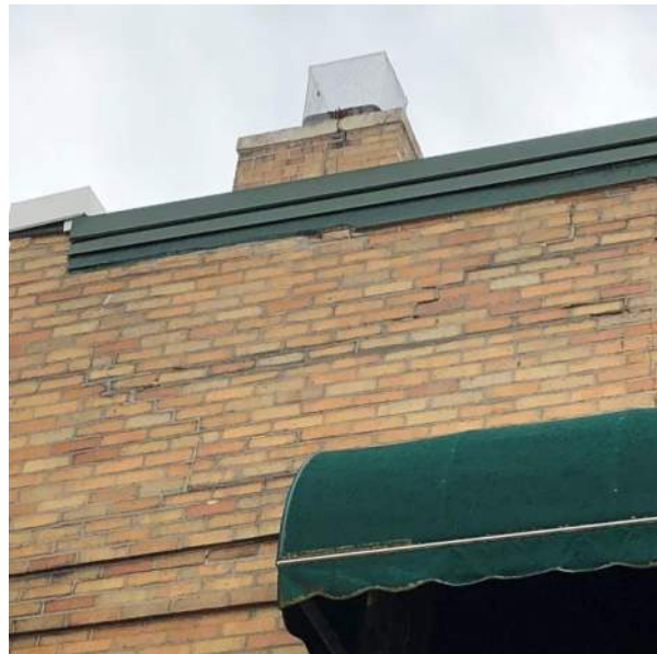
B-v: Failing Brick
