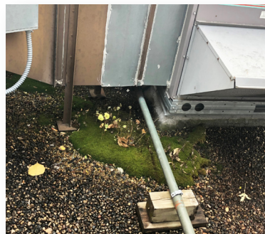
Vegetation grows in standing water on the roof.
