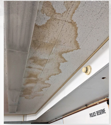
Water damage from roof and wall leakage is prolific throughout the building, in some cases leading to visible mold growth.
