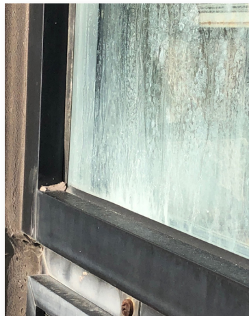
Water intrusion has permanently damaged most building windows.
