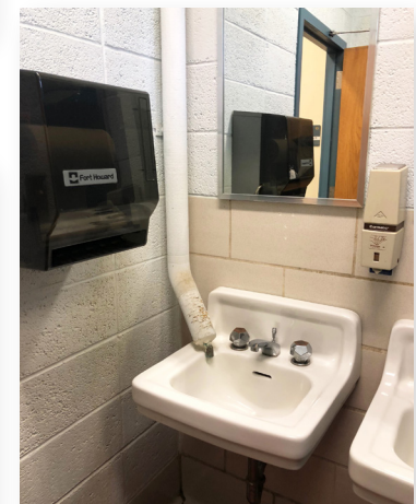
A pipe wrapped in asbestos drains into an employee bathroom sink.
