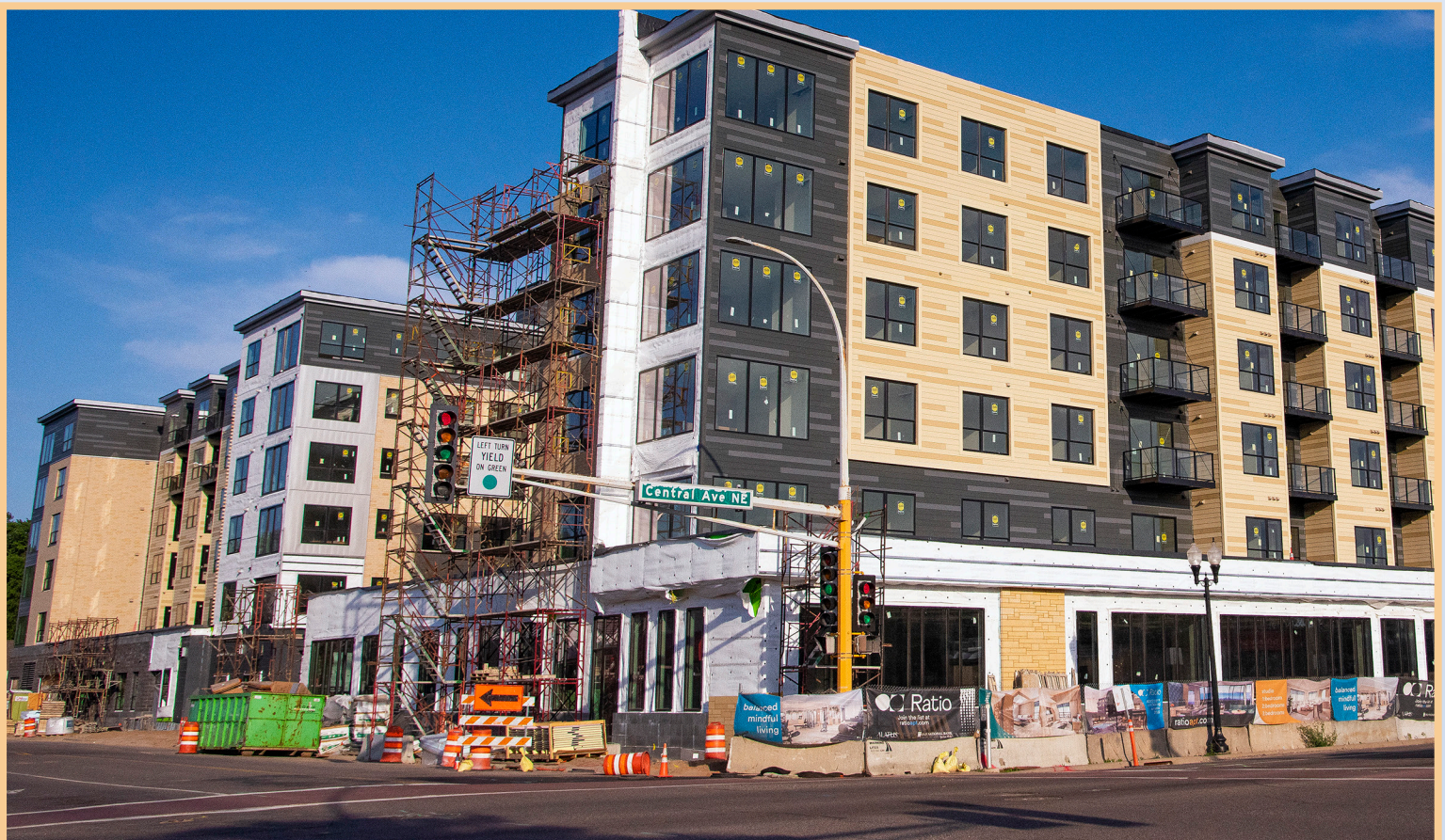
Above: The New City Hall and Ratio Apartments under construction in 2022.
