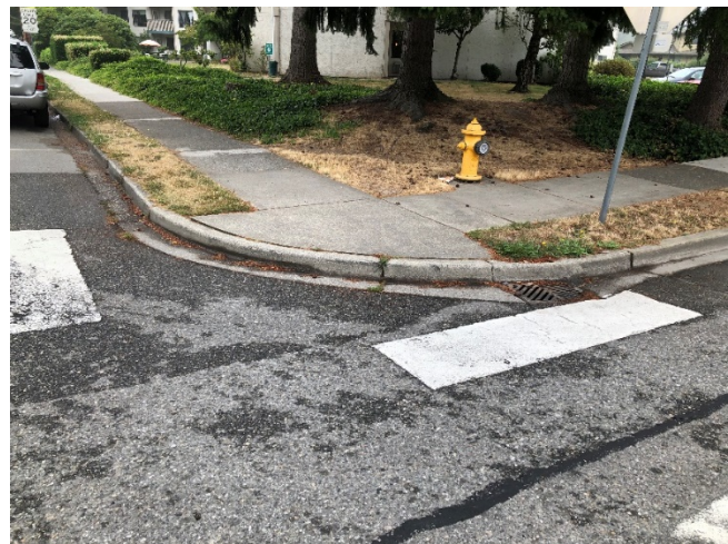
ADA Barriers include missing curb ramps at crosswalks such as these at the intersection of State Street and Township Street.
