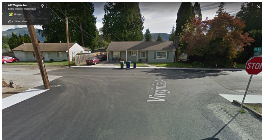
Figure 16. Lack of Detectable Warning Surface and Fixed Object at 677 Virginia Ave.
