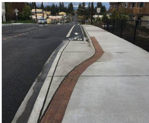
Figure 1. Sample ADA Roundabout Detectable Edge Treatment at Bicycle Ramp
