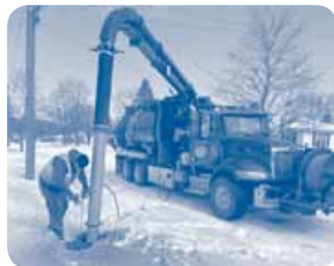
Locating customer service lines to verify material type. All lead and galvanized service lines in the State of Michigan will be replaced by local water systems in the coming years.
