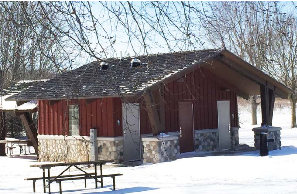
River Cobble and Wood Slat Restroom This restroom facility features wood slats with a river cobble base. The roof overhang extends to cover the entrances into the men's and women's restrooms. A metal roof would be preferable to the shingled roof shown in this image. It also features a more square layout, with the men's and women's restrooms being back-to-back.
