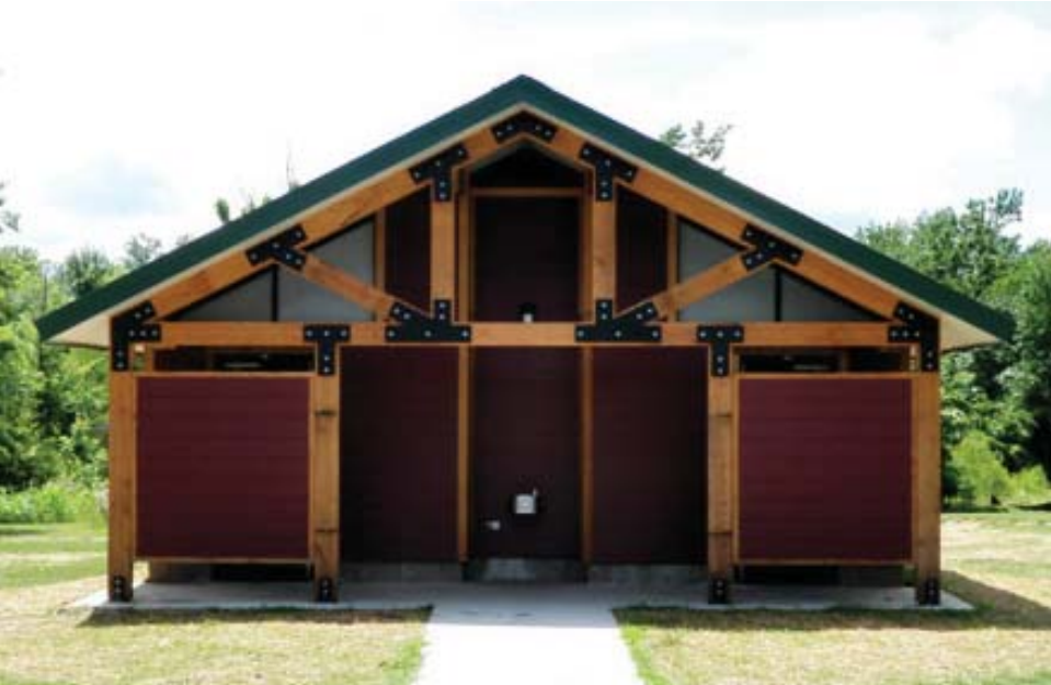
Screened Restroom Entrances This restroom is comprised of wood posts and beams and wood siding. The entrances to the men's and women's restrooms are screened, which might be preferable as it reduces visibility from the outside into the restrooms. It features a more square layout, with the men's and women's restrooms being back-to-back.
