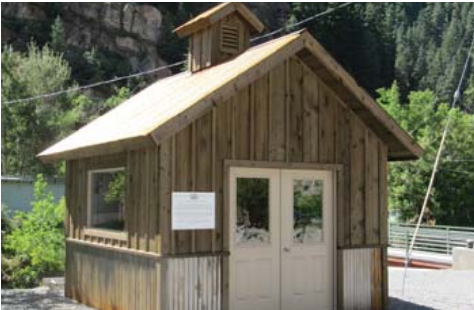
Micro-Hydro Building (Materials Precedent) This existing Micro-Hydro building by the Ouray Hot Springs is another example of the types of materials that would be featured in the proposed new stage and restroom facilities. This structure features corrugated steel roofing and wainscoting (not treated so it will weather) and wooden siding to promote Ouray's mining history.
