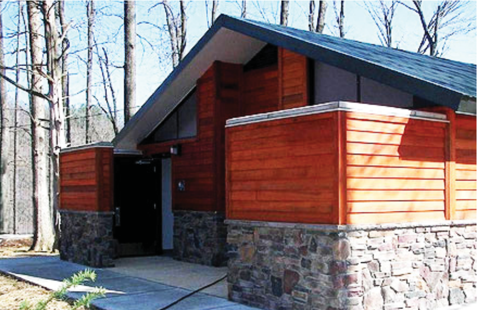
Screened Restroom Entrances with Stone and Wood The screened entrances on these restrooms are sturdier and conceal more than in the image shown to the left. The stone base of the structure partnered with the wood siding would complement the different natural materials found in Ouray.
