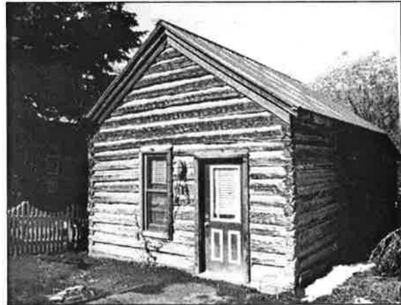
Pioneer Log Building at 318 Main Street (5OR.585.14) 2004 by Grant Houston.
